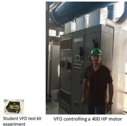
**Figure 3. (Left) Small 1HP VFD test kit, (Right) VFD controlling a 400 HP motor**
